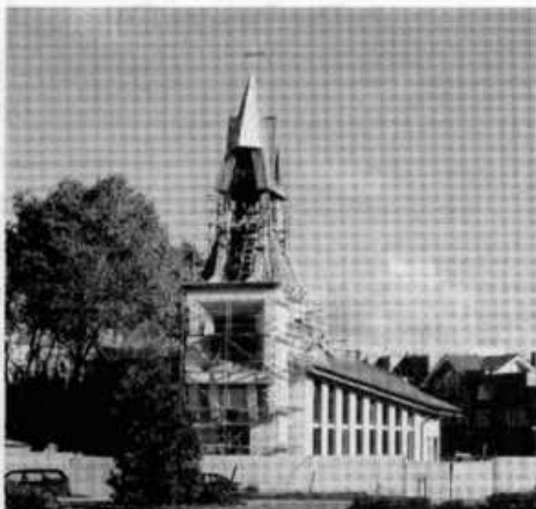
Palanga church and diaconical center under construction
