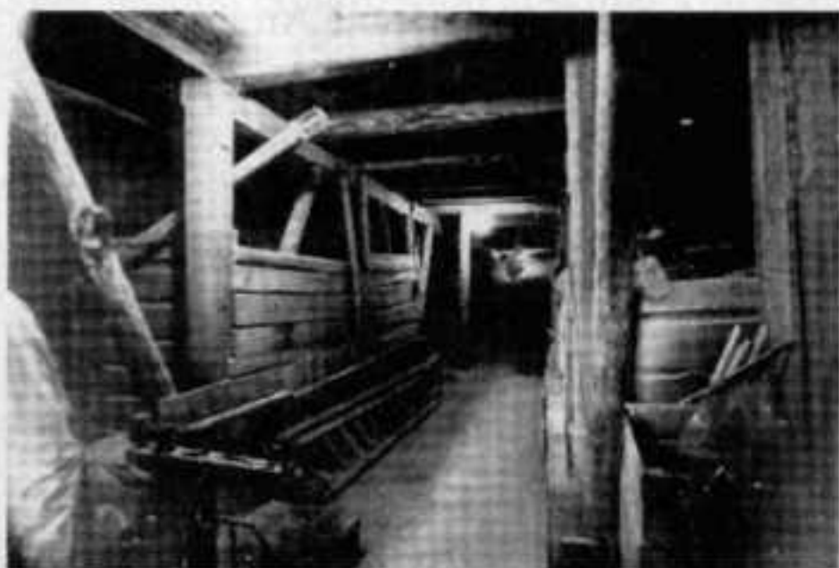
Dovilai church used to store grain, 1988
